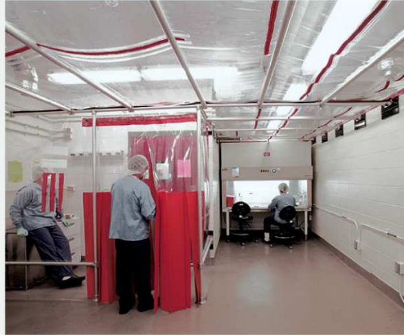
Architecturally Renovated Containment Room
